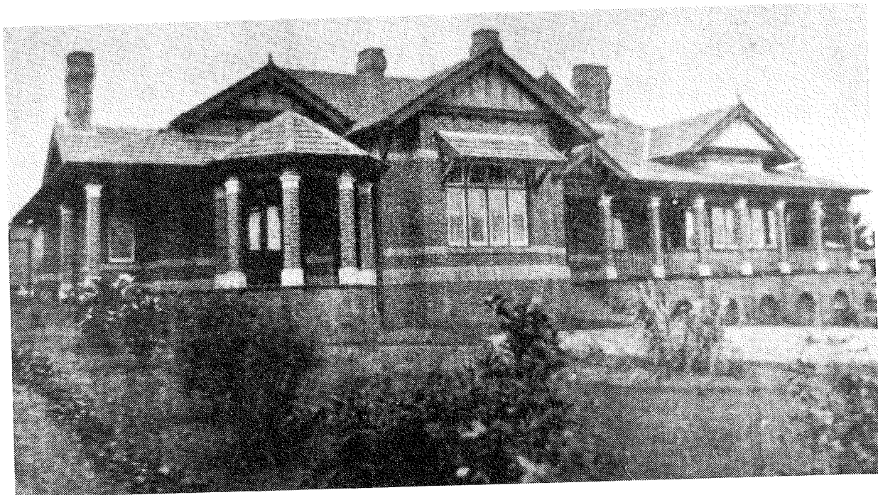
Mr W J Clarke's Residence, Clendon Road, Toorak, Beverley & Ussher, architect, (B.E.&M.J. 4.12.1897)
