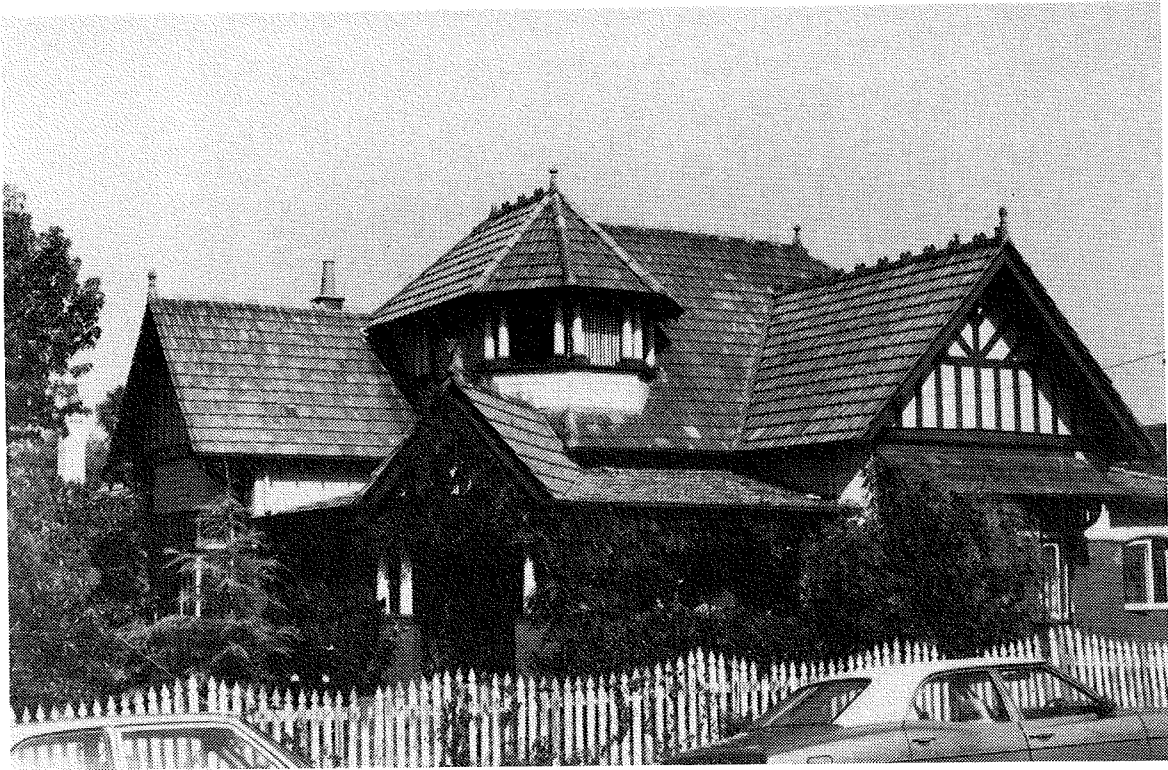
40 Christobel Crescent, Hawthorn; Christopher Cowper, architect.
