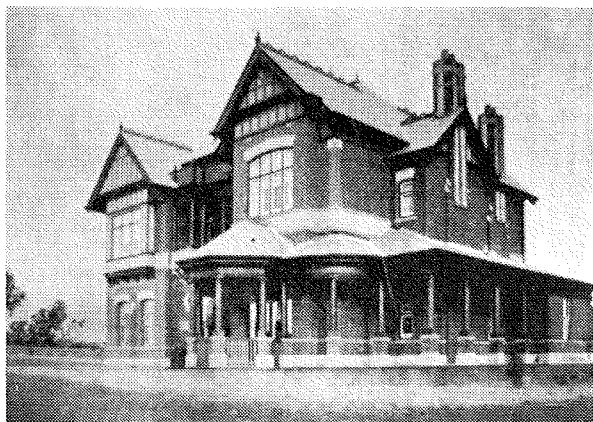
Residence, Canterbury, Beverley Ussher, architect (B.E. & M.J., 27.11.1897)
